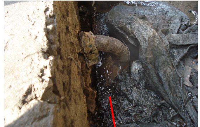
After TLV Trap installation
